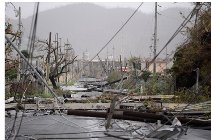
Puerto Rico after Hurricane Maria
